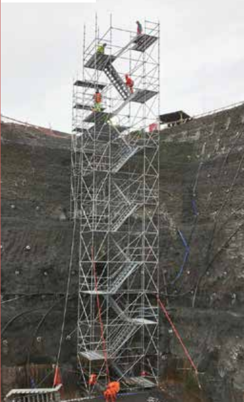
19 Torre escala industrial
